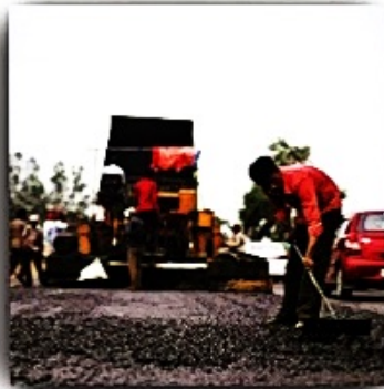
Road Construction (Urban, Rural, PMGSY)
