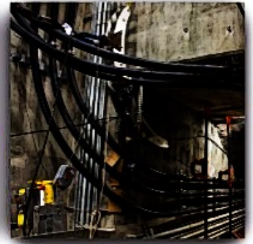
Power Cabling & Electrification Works
